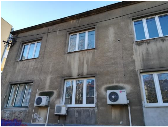
Figure 3. a) Inadequate sill solution on a masonry structure ( https://pxhere.com/en/photo/779893 ); b) inadequate air-conditioning
